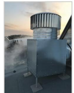
Ecopower allows natural ventilation during the day to meet or exceed minimum outdoor air ventilation rates requirements of ASHRAE standard 62.1. The powered mode can be activated at night by a timer or temperature sensor. The night purge operation removes excess heat in the room or building allowing cool night air to reduce the stored energy and cool the building down. This reduces daytime cooling loads and lowers energy consumption.
