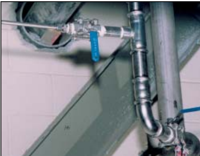
The Pressfit system provides unparalleled versatility. With a variety of o-rings for most applications, Pressfit system components provide reliable, leak-free service. This instrumentation line was installed more quickly and economically when compared to other traditional joining methods.
