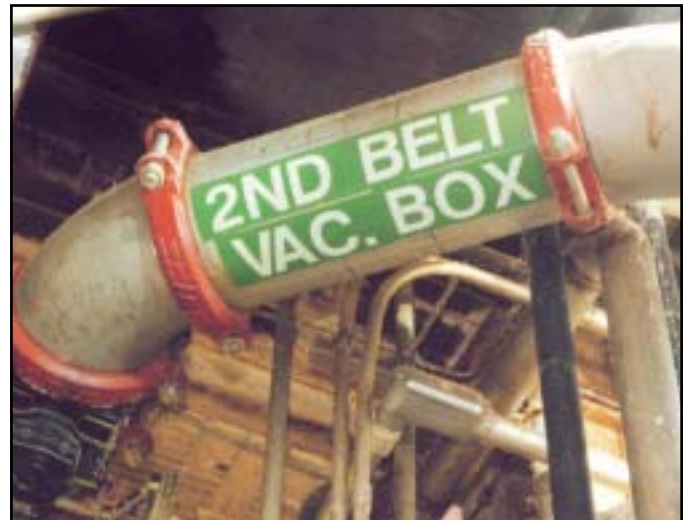
The grooved system remains the fastest method for joining 2 through 12-inch (50 - 300 mm) stainless steel piping systems. Requiring just two bolts and nuts to complete a joint, the Victaulic system can reduce your installation time by 30 - 50%.
