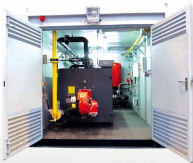
Gas fired Hot Water Plant Room
